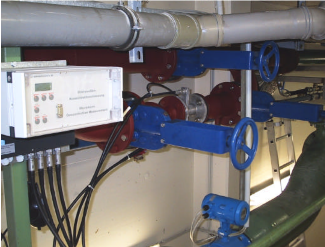
Abb. 4: Installed measuring system: Measuring cell in a bypass pipeline connected with a high frequency cable with the evaluation unit Micro-Fluid LB 455, sewage treatment plant, Gütersloh
